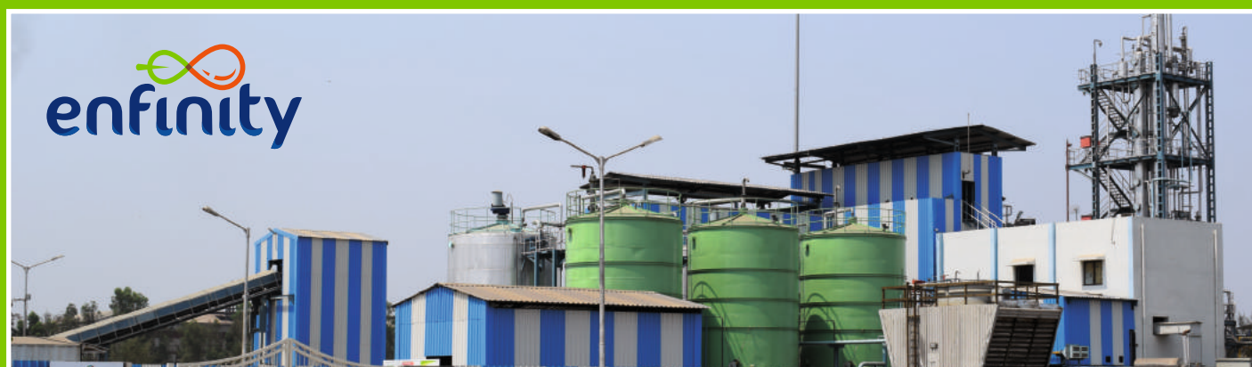
Praj's Integrated 2 nd Generation Smart Bio-Refinery Demonstration Plant
